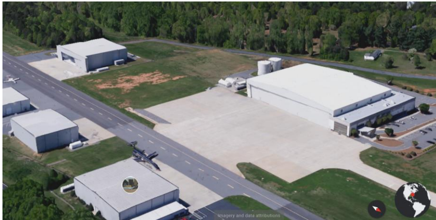
Jet East facility in Statesville, NC
